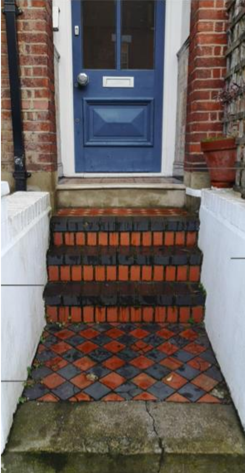
1. Existing Site: front door, glazing and steps arrangement
