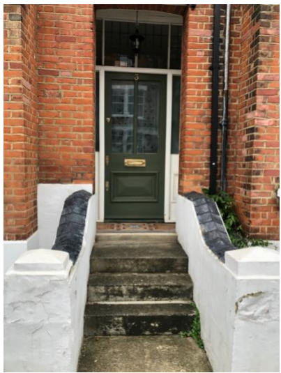
2. Off site: Front door and glazing arrangements showing plain and leaded examples. Top landing decorative tiles appear as part of the character of the conservation area (CA).
