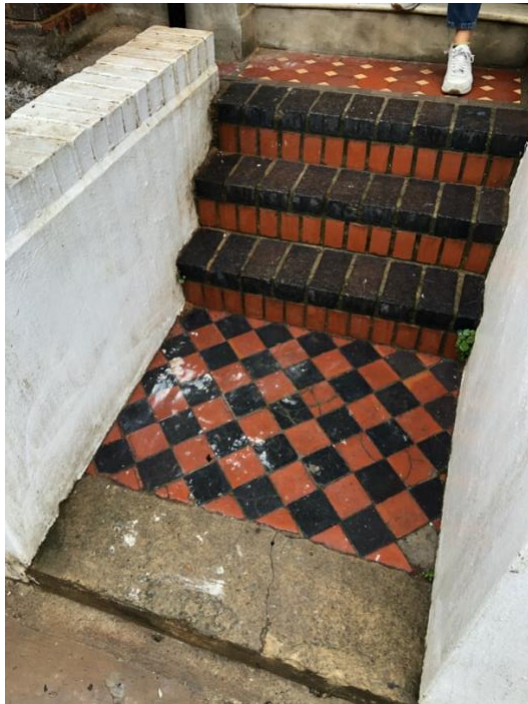
6. Existing site: front steps and landings.
