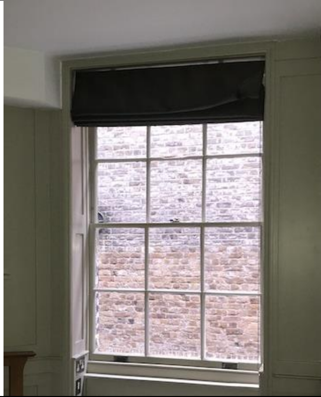
Second floor (rear elevation)
