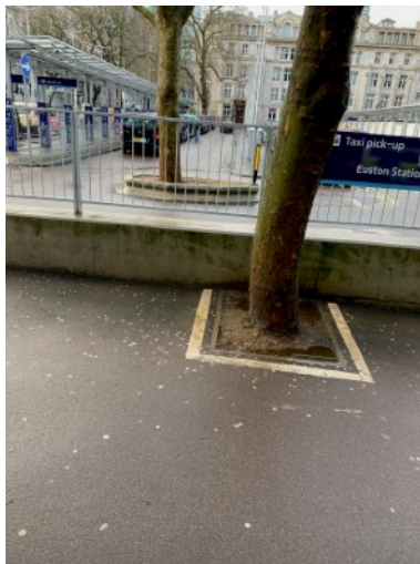
Nearby trees surrounded by asphalt
