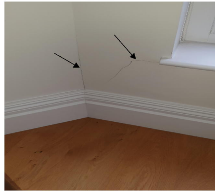
Crack to bay in flat 28
