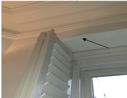
Crack to bay area of flat 26.
