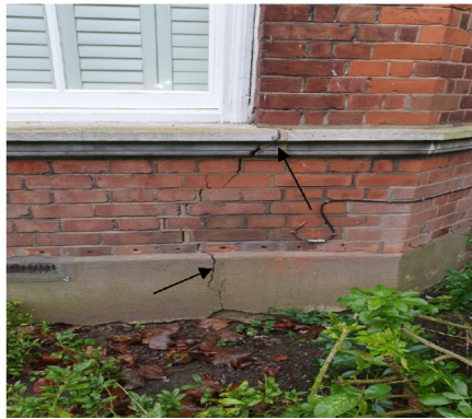
Cracking to ground floor bay (Right Elevation)
