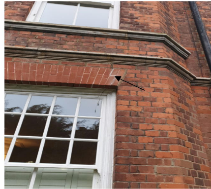
Cracking to first floor bay (Right Elevation)
