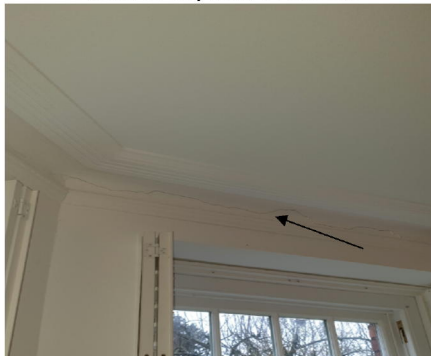
Crack to bay and cornice flat 26.
