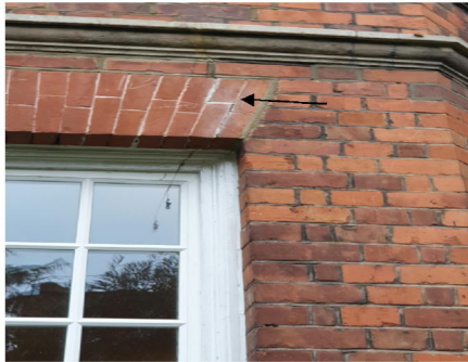
Close up of cracking to first floor bay (Right Elevation)
