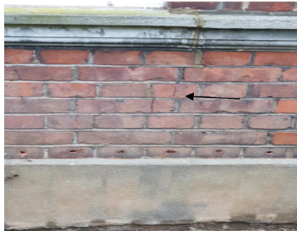
Cracking to ground floor bay (Front Elevation)
