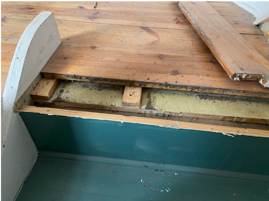
Existing Pine Flooring at Ground Floor level
