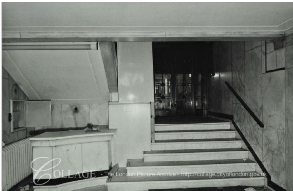
Figure 1. View of entrance lobby, note solid wall seen to the right of the image and timber and glazed partition beyond. The amended proposal can therefore be understood to be a reinstatement of a historic partition which is illustrative of the original use of the space.
