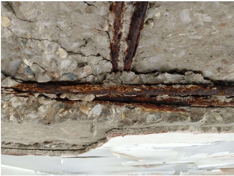
Site photo of corrosion to existing steel bars
