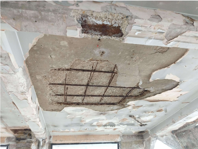
Site photo of slab soffit following loose concrete removal. Many bars have suffered significant corrosion due to suspected water ingress.
