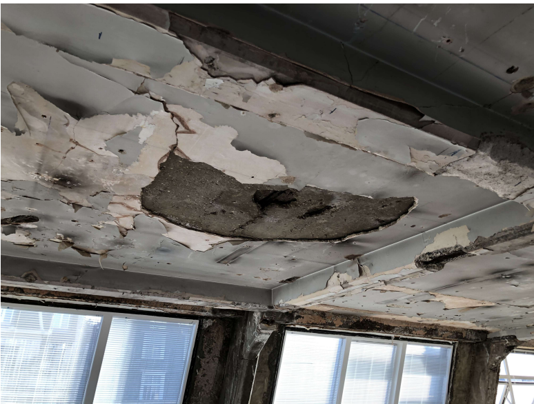
Site photo of condition following soft strip. All loose concrete was removed due to health and safety and to inspect the condition of the remaining slab
