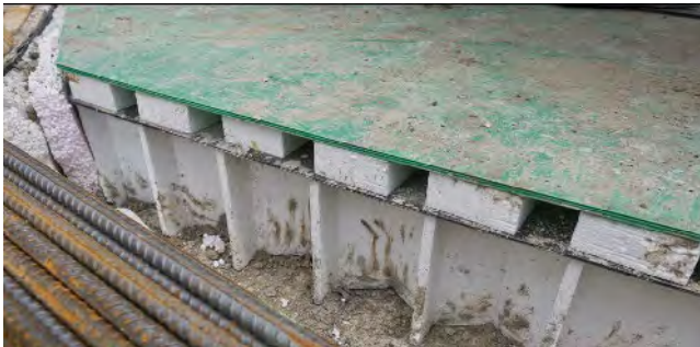
CORDEK Cellvent laid on heave protection
