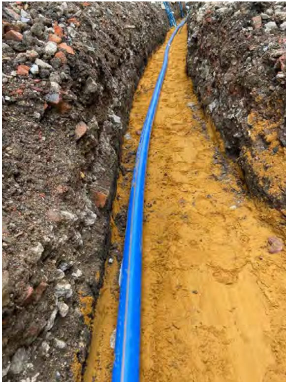
SITE PHOTO SHOWING BARRIER PIPE BEING INSTALLED
