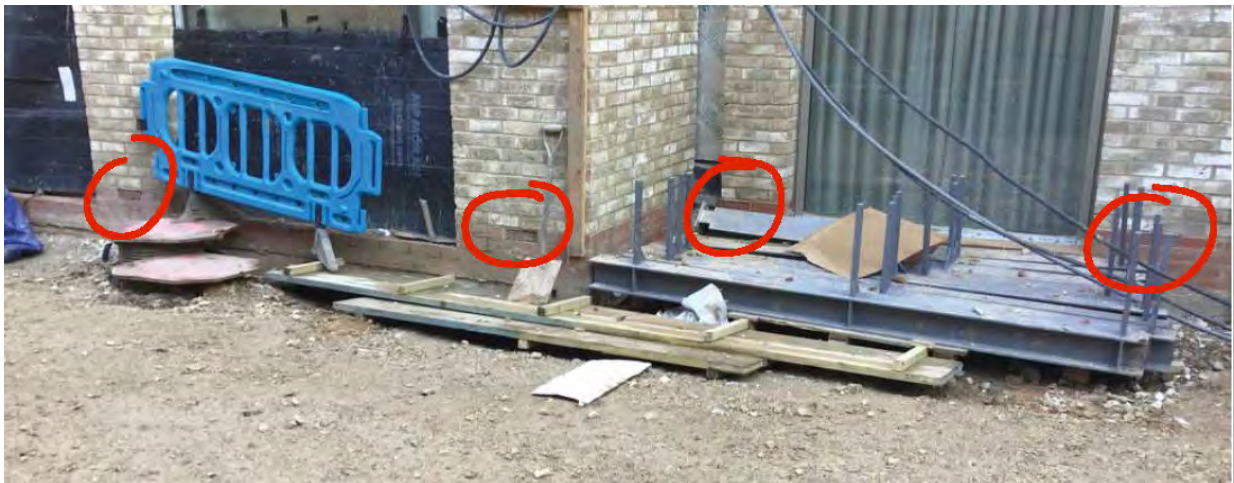
SUB-FLOOR VENTILATION POINTS
