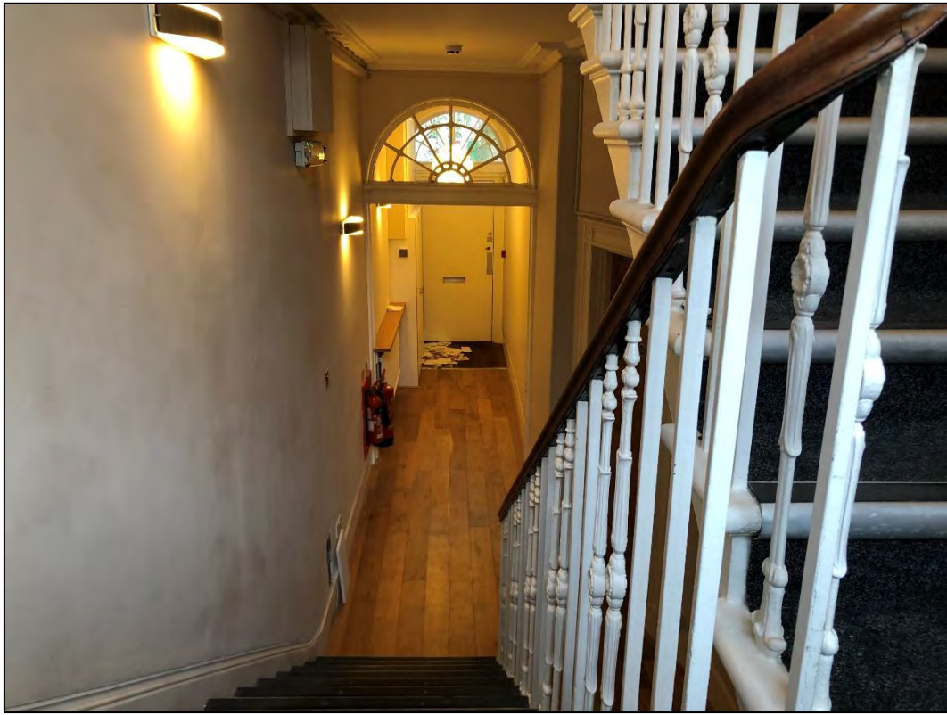
Plate 13: View showing detail of staircase to first floor with mahogany handrail and wrought-iron balusters
