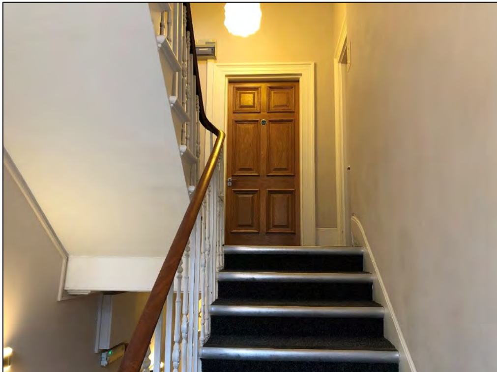
Plate 13: View showing detail of staircase to first floor with mahogany handrail and wrought-iron balusters
