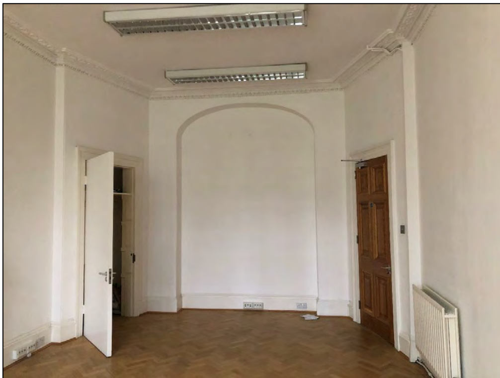
Plate 7: View looking W showing blocked archway in W wall of ground floor front room
