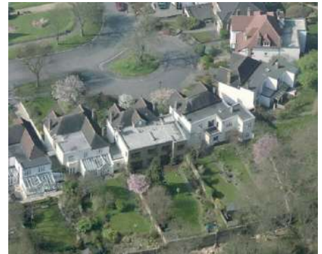
Rear aerial view of site
