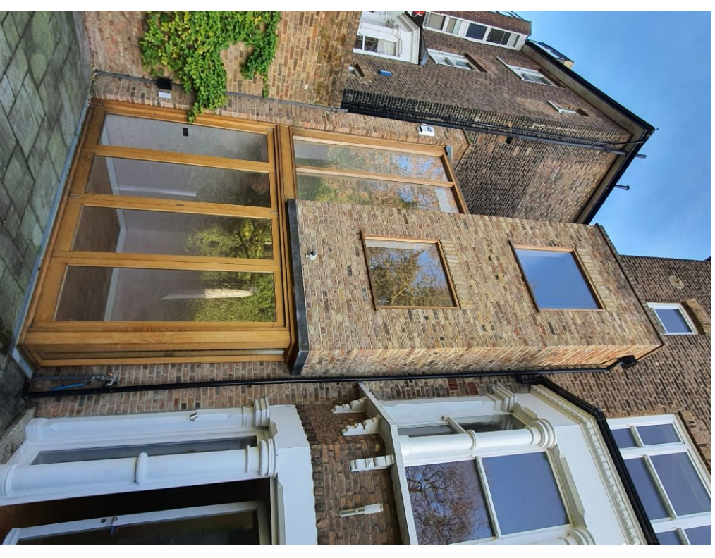
Existing rear and side extension
