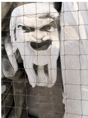
Figure 6 photos showing gypsum crusts
