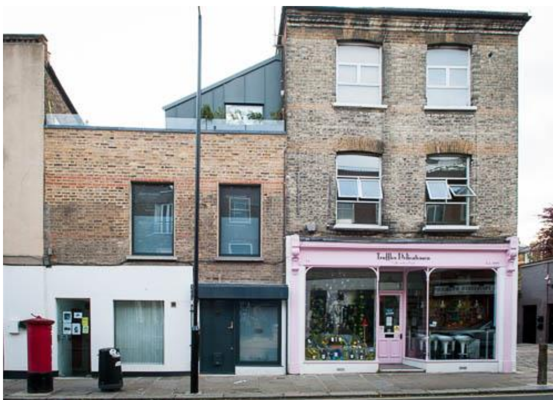
Roof extension, York Rise
