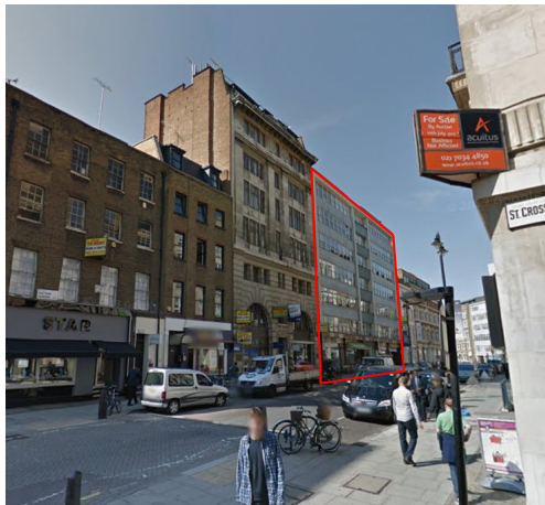
View of the existing building from the South
