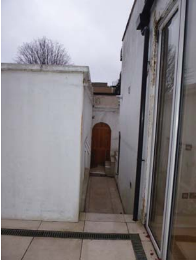
View from rear garden to side entrance
