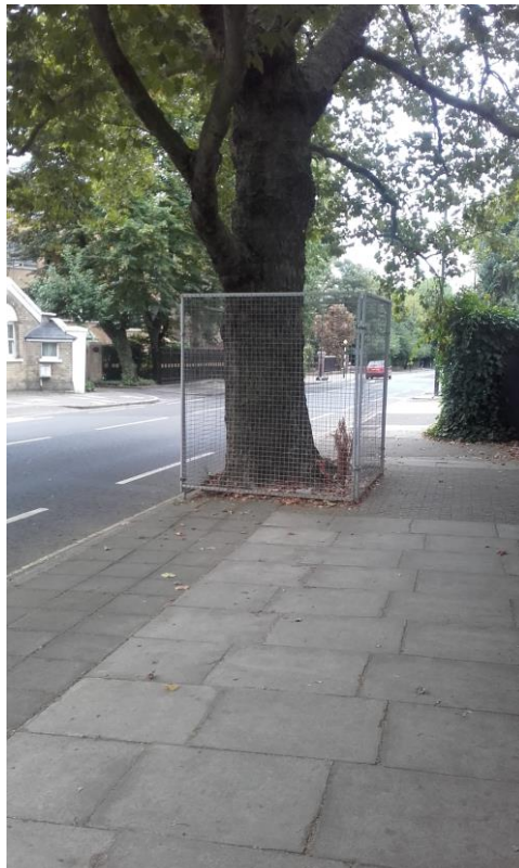
Image 4 - Protective fencing, stem protection caging: Where space allows, larger tree stems can be protected using metal cages. It is necessary to secure the mesh panels to the ground using screwed fixings.
