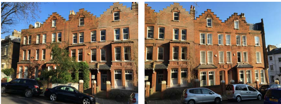
The residential terraced row 2-14 Well Walk in Hampstead with its distinct stepped gable and red brick. No 8 is located in the middle of the row.
