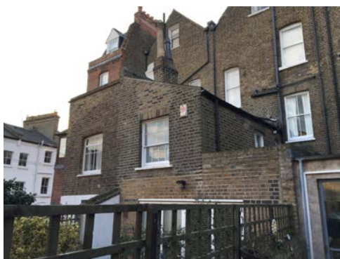
View towards altered rear elevations to the South.
