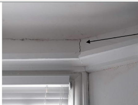
Photograph 15 Front LHS bedroom – above bay window
