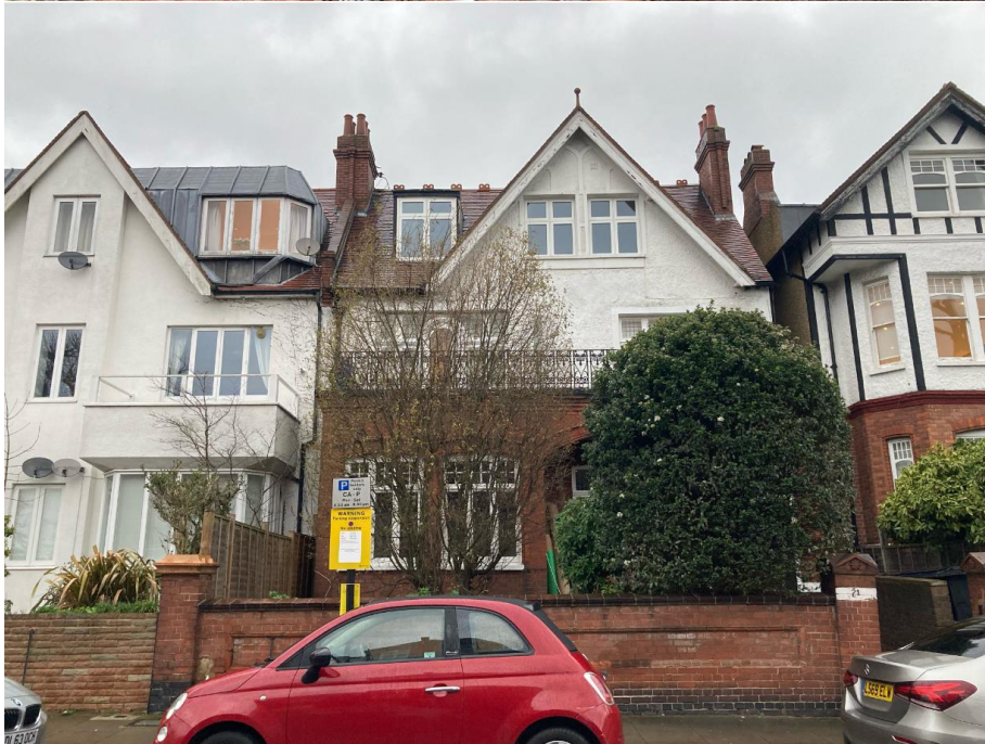
Above: Photos of front elevation
