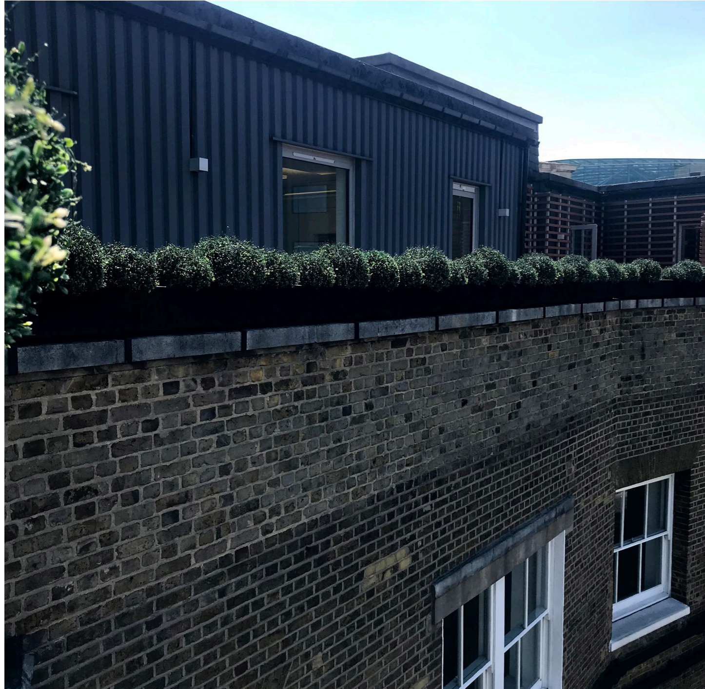
Existing parapet back elevation of 4th floor with non original brick parapet to be removed
