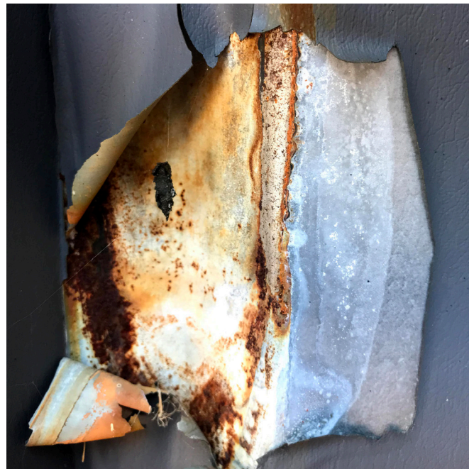
Aged cladding dilapidated and rusting
