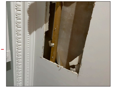
Typical dropped modern plasterboard ceilings
