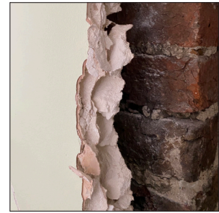
Modern Plasterboard on dab & dot
