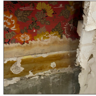
Modern Plasterboard on dab & dot
