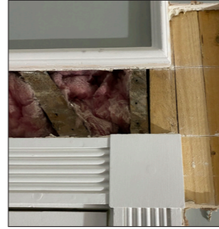
Internal modern plasterboard on timber stud with modern insulation
