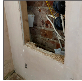
Modern plasterboard on timber stud brick spine wall behind
