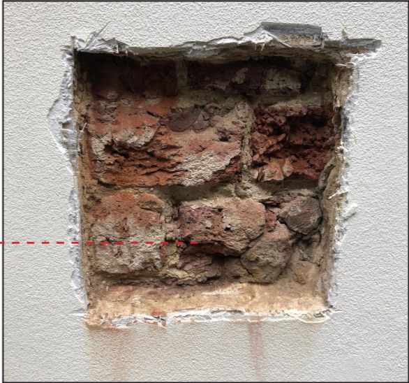
Detail of External Render Intrusive Survey
