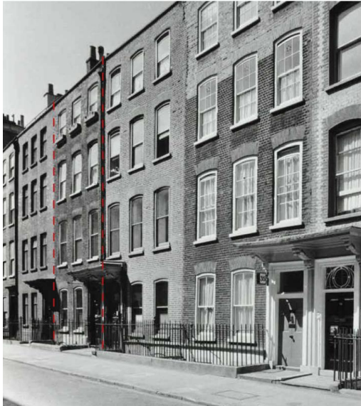
Figures 2: A general view of four-storey buildings at 38-34 Great James Street
