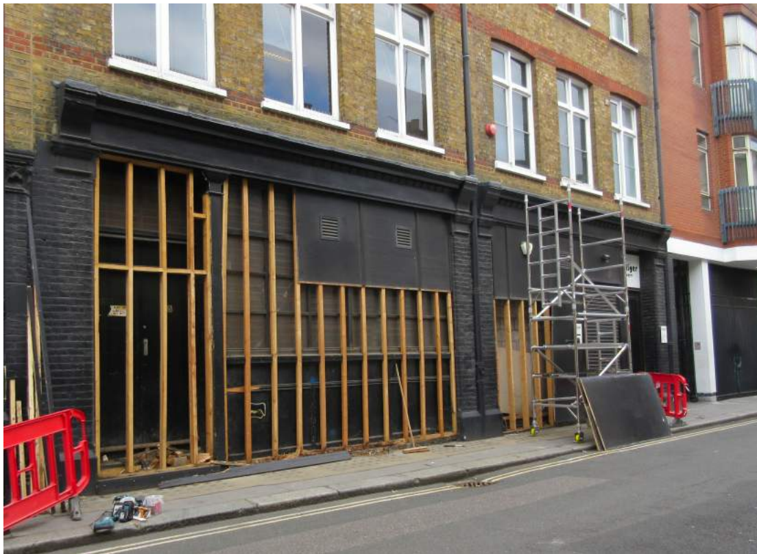
Figure 3: Existing shopfronts at Nos. 2 (right) and 3 Morwell Street
