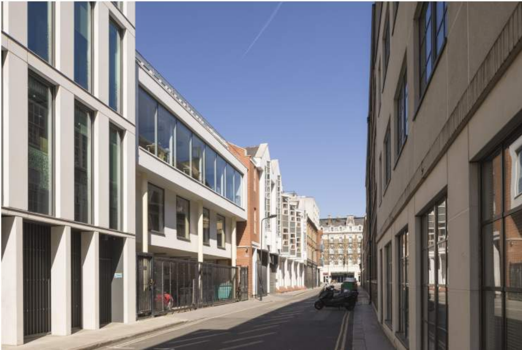
Figure 9: Existing view looking north along Morwell Street
