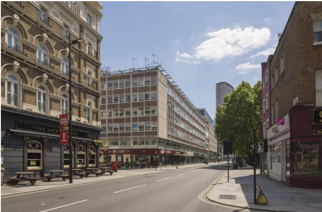
Figure 11: Existing view looking south along Tottenham Court Road.
