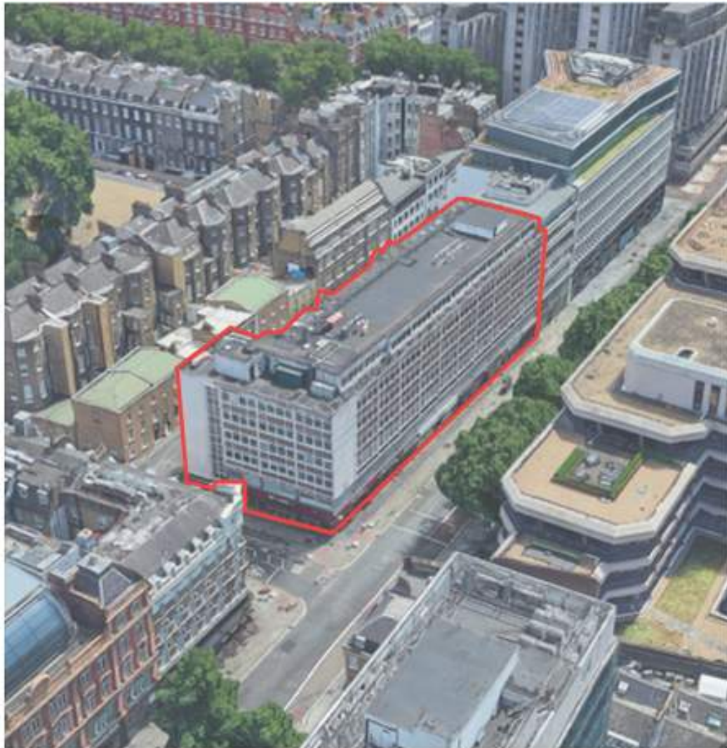
AERIAL VIEW LOOKING SOUTH EAST
