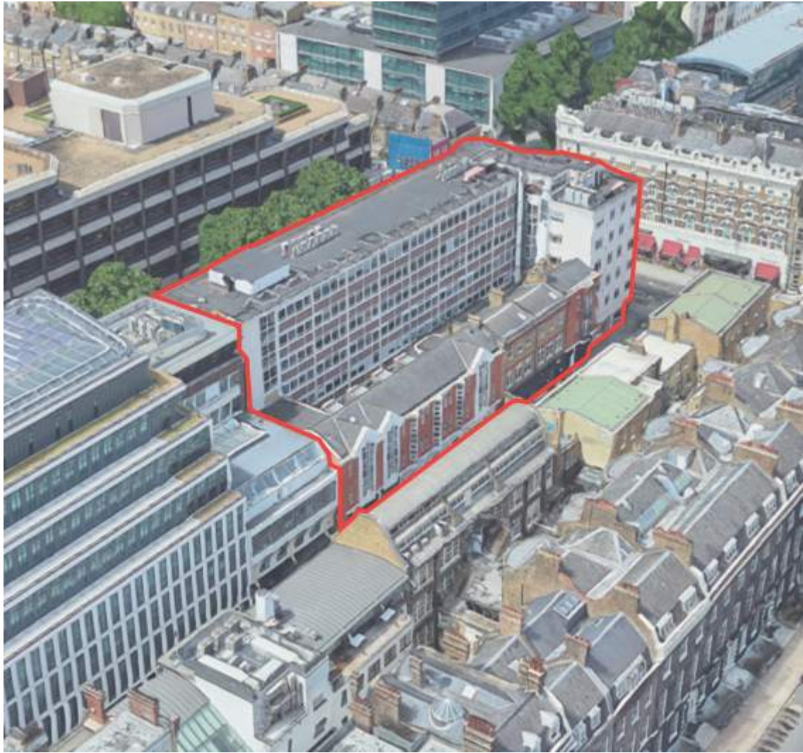
Figure 13: Existing buildings on site viewed from the south
