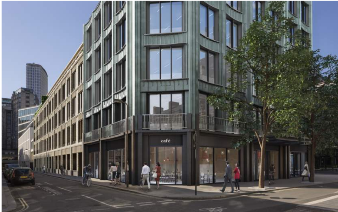
Figure 15: View south along Morwell Street
