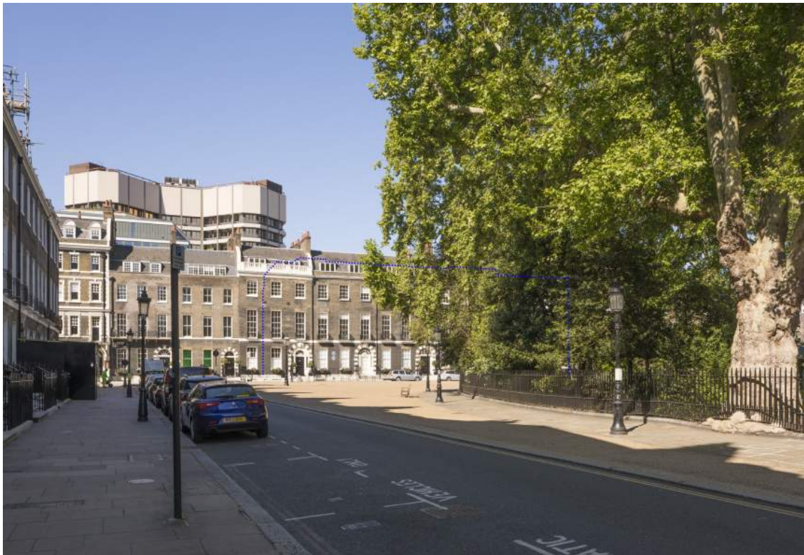
Figure 8: View 9 looking west along the northern edge of Bedford Square.
