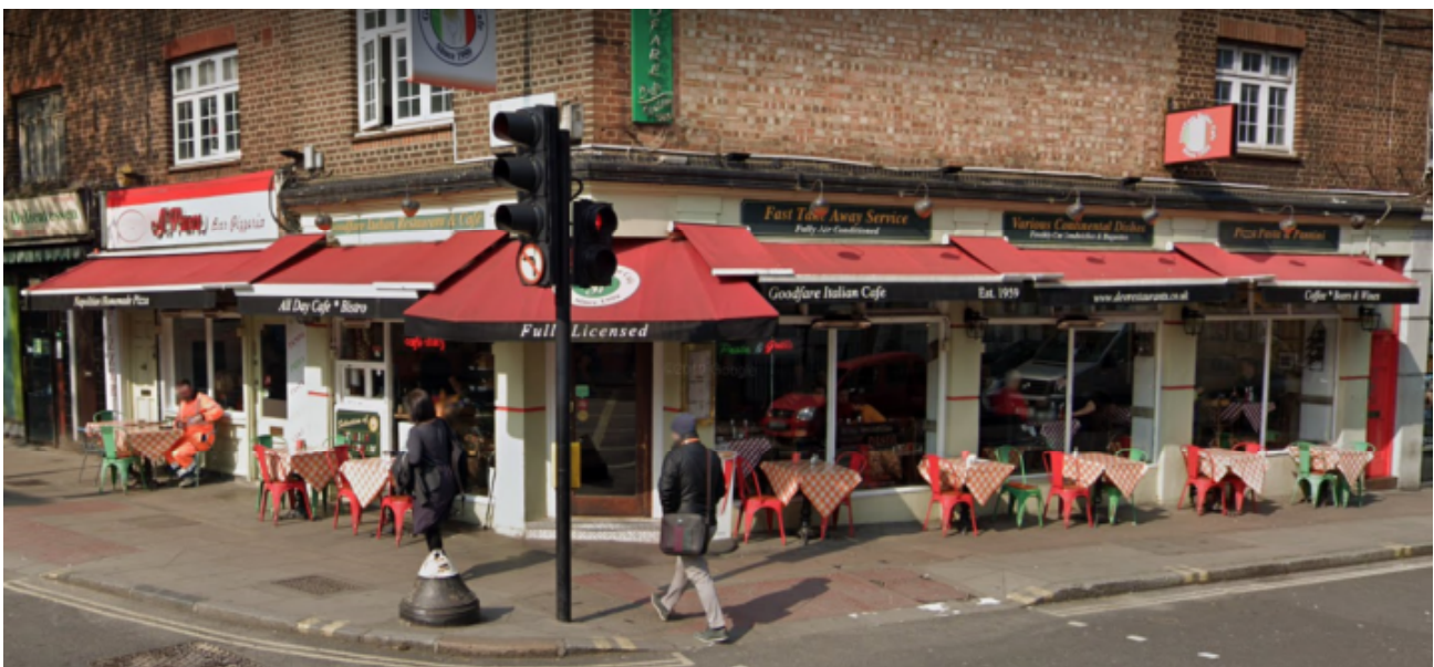
Photograph 1: showing application site (26-28 Parkway)
