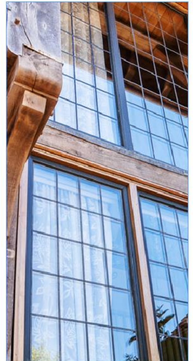
ARCHITECTURAL BRONZE CASEMENTS Example showing applied lead to conservation double glazed unit.
