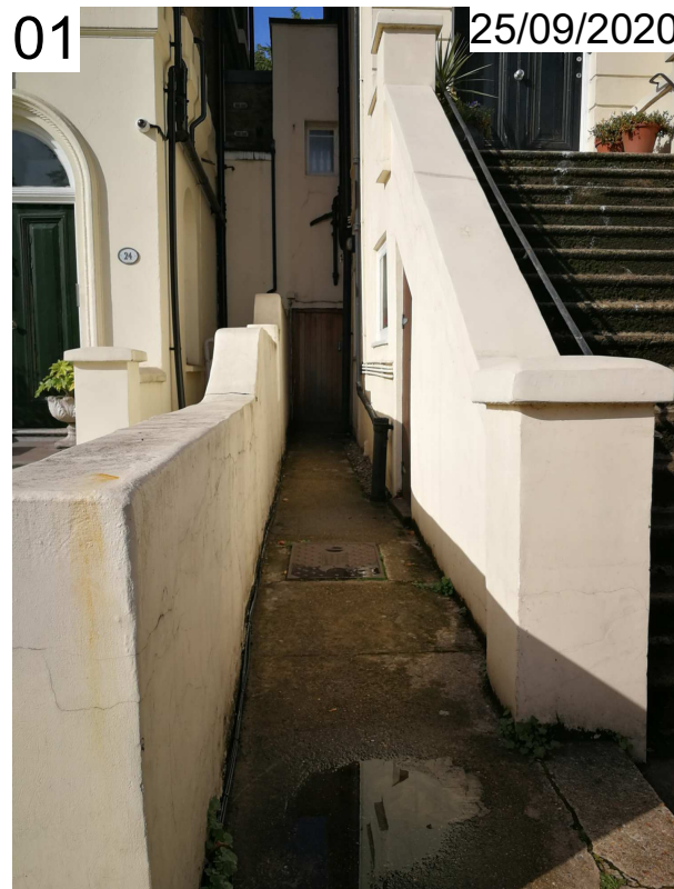
- No.25A Entrance access walkway.
