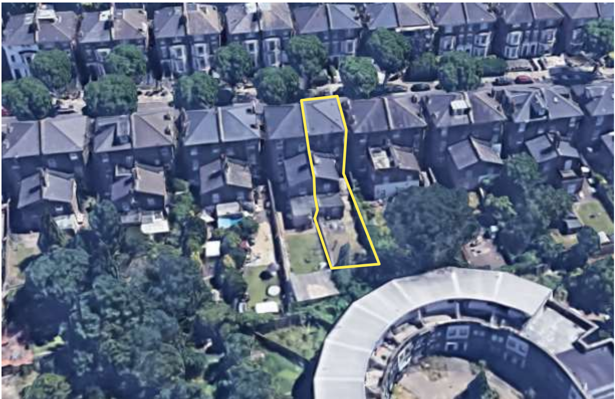
Aerial view of rear elevation (Site outlined in yellow, Google maps)
