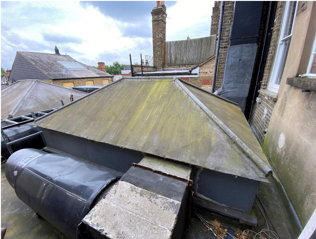
IMAGE 1: PRE-EXISTING CONCRETE BOARD ROOF AND DUCT
