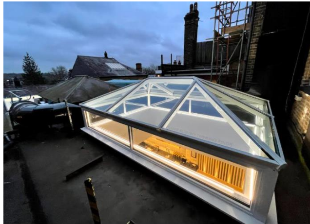
Image 3: Roof lantern in-situ
