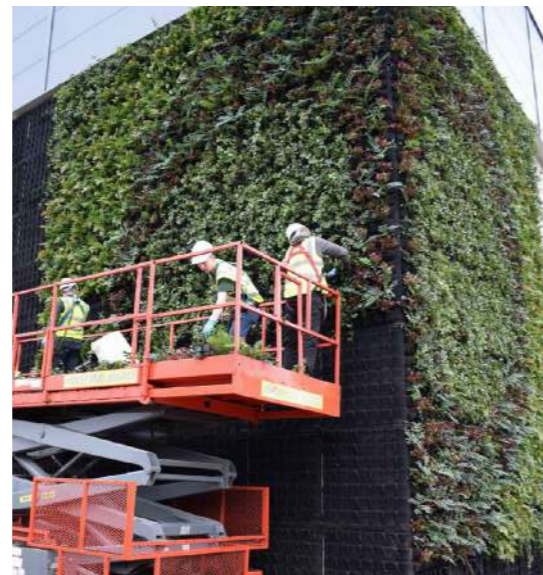
Living Wall constructed with Fytotextile
