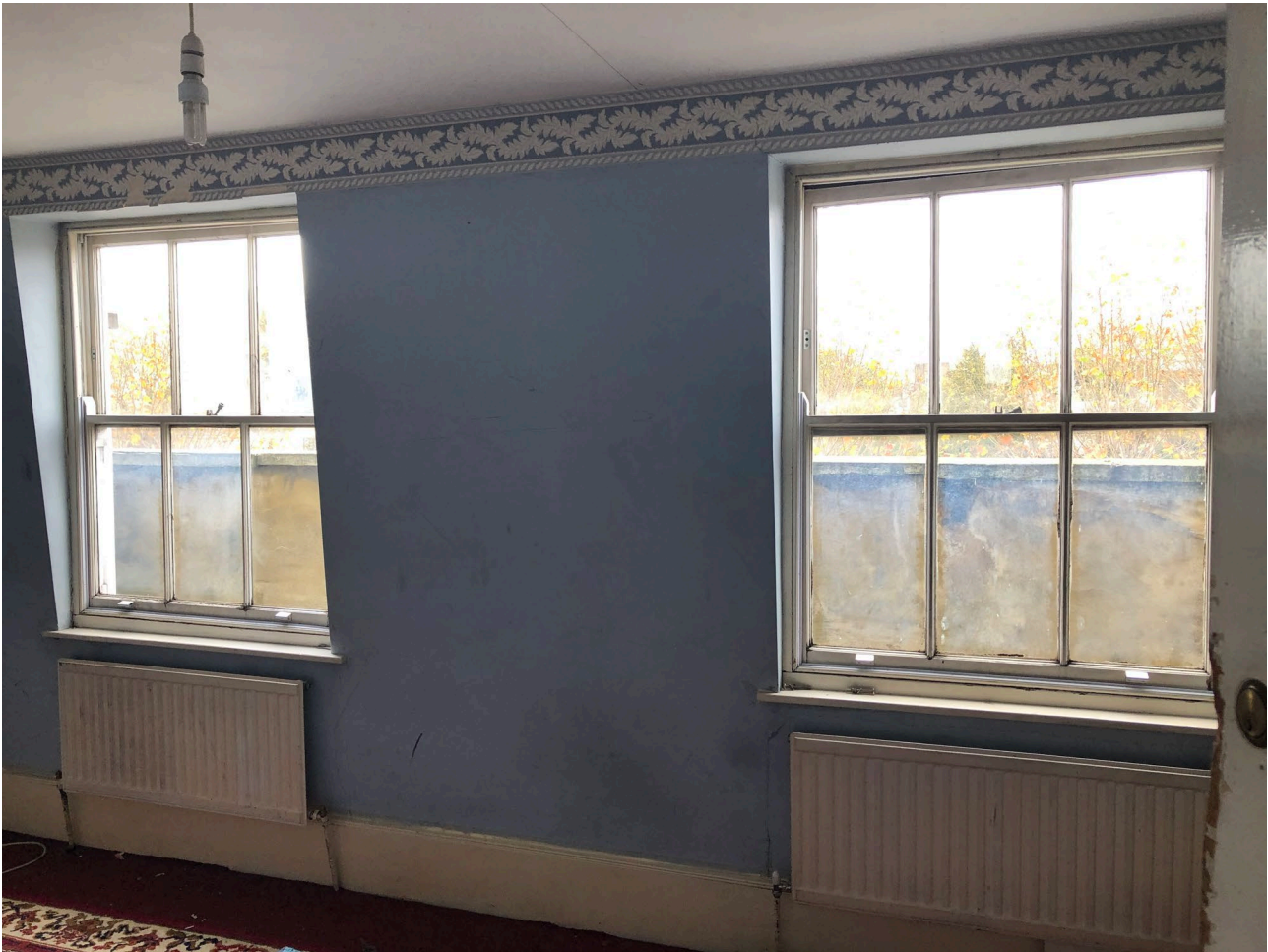
Figure 5: Internal view of bedroom windows at third floor level (Flat C)
