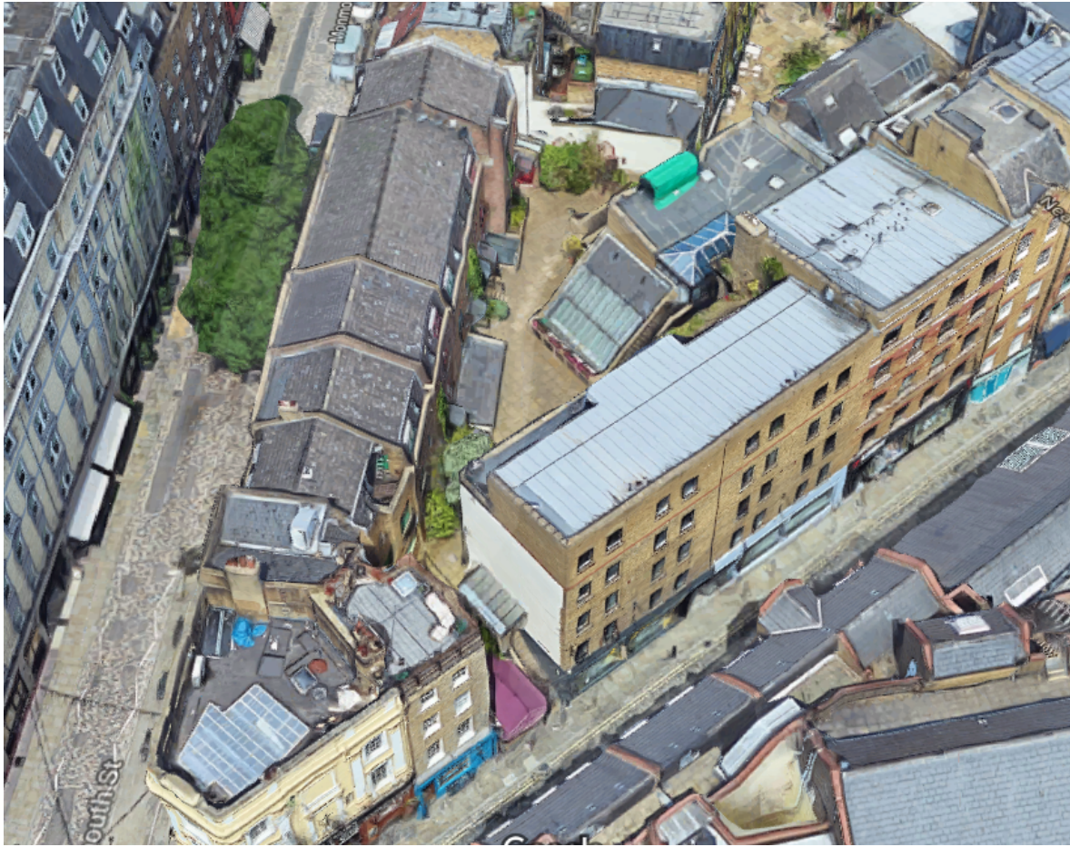
Photo 1 (above): Aerial view of site. Existing plant on roof is visible covered by a green tarpaulin
