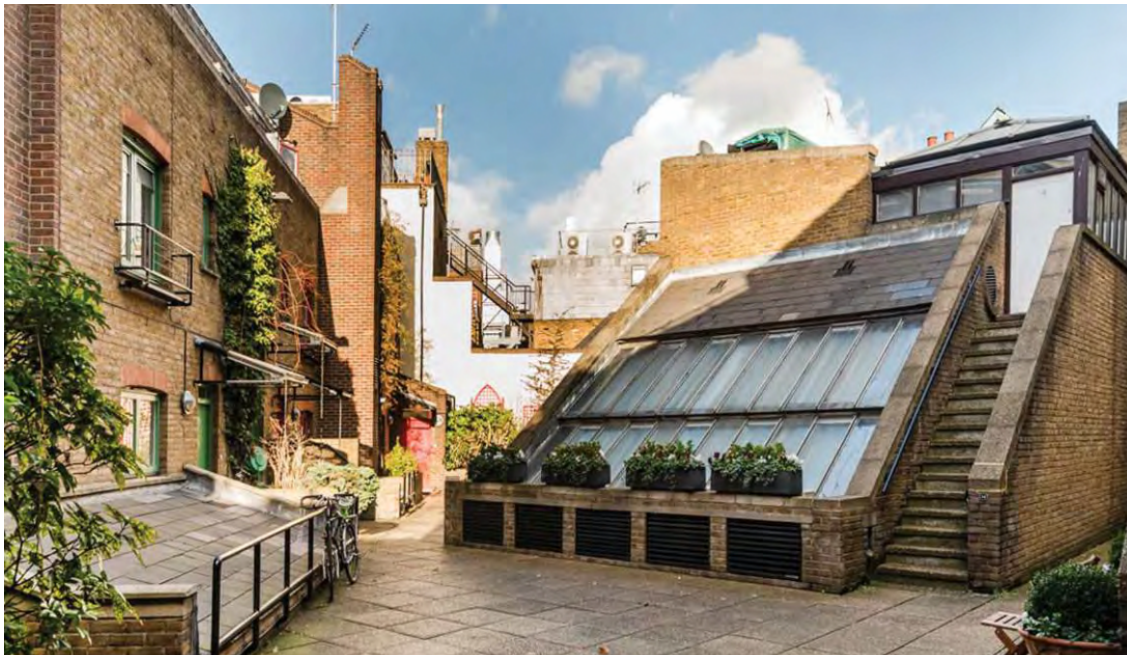
Photo 2 (above): Courtyard of Seven Dials Court looking north-east towards Neal's Yard. The existing plant on the roof can be seen covered by a green tarpaulin.
