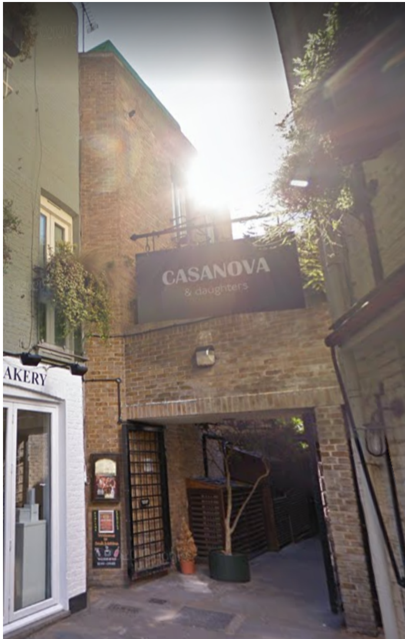
Photo 4 (above): North elevation of site adjacent to 3 Neal's Yard to which the linear access panels would be installed
