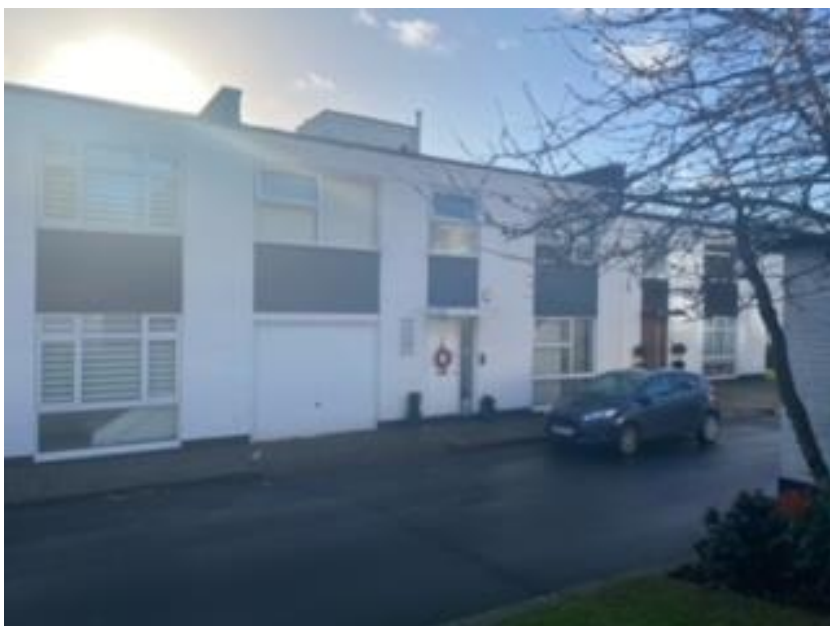
Photo 3 (above): Front elevation of Nos. 17-13 Hawtrey Road
