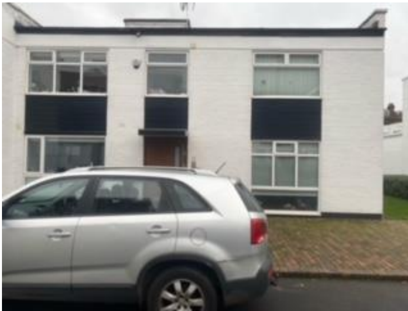
Photo 1 (above): Front elevation of 13 Hawtrey Road
