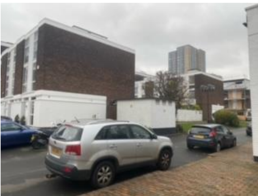
Photo 6 (above): Front and side elevation of 82 Hawtrey Road opposite No. 13
