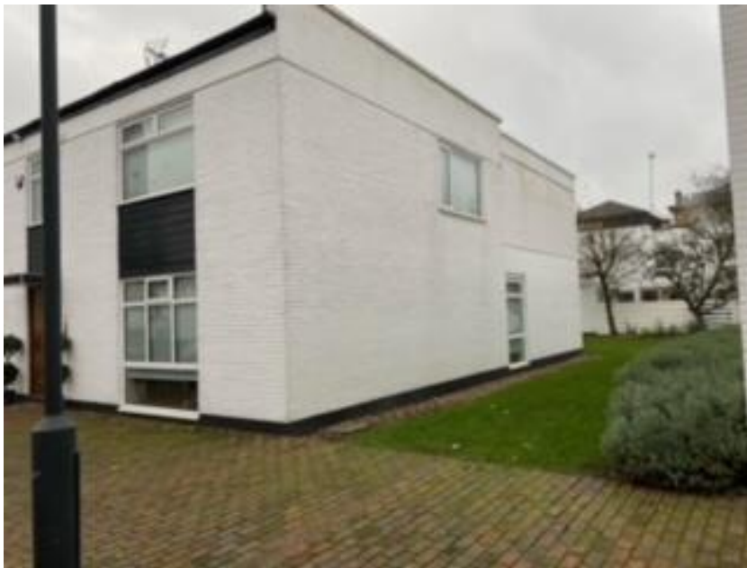
Photo 7 (above): Front and side elevation of 13 Hawtrey Road and adjacent communal garden
