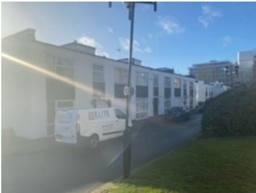
Photo 2 (above): Front elevation of Nos. 19-15 (odd) Hawtrey Road
