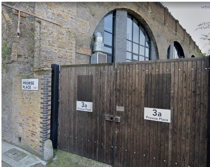
Figure 6.1: Existing Air Handling Units
