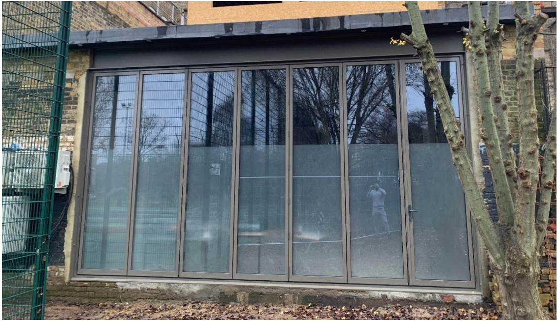
Picture 12: External view of bi-folding doors (Master door to furthest right)
