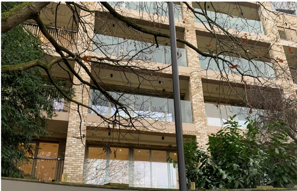
Picture 15: Modern floor to ceiling glazed doors to rear elevation overlooking Kilburn Grange Park
