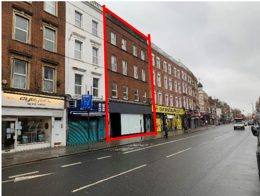
Picture 1: South View down Kilburn High Road – 292-294 ‘the property’ outlined in red
