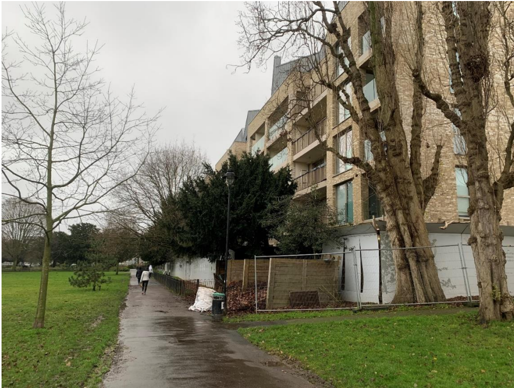
Picture 14: Newly built local modern 6-storey development overlooking Kilburn Grange Park
