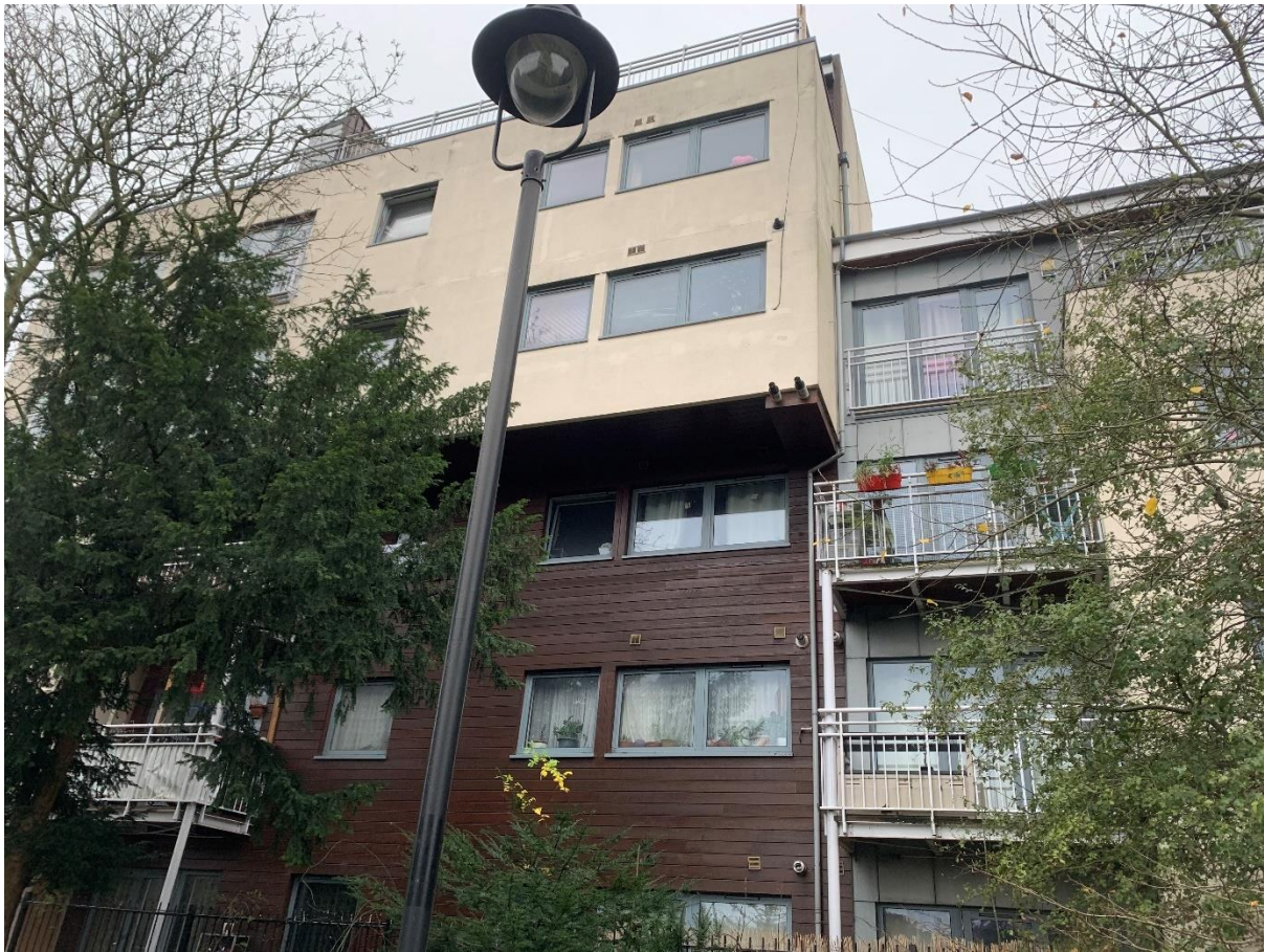
Picture 17: Local modern build overlooking Kilburn Grange Park – rear boundary 2m off pedestrian footpath
