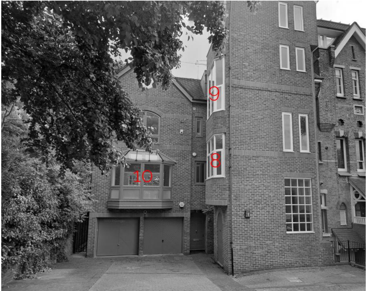
Above – Windows 8 to 10 at 7-9 Prince Arthur Road
