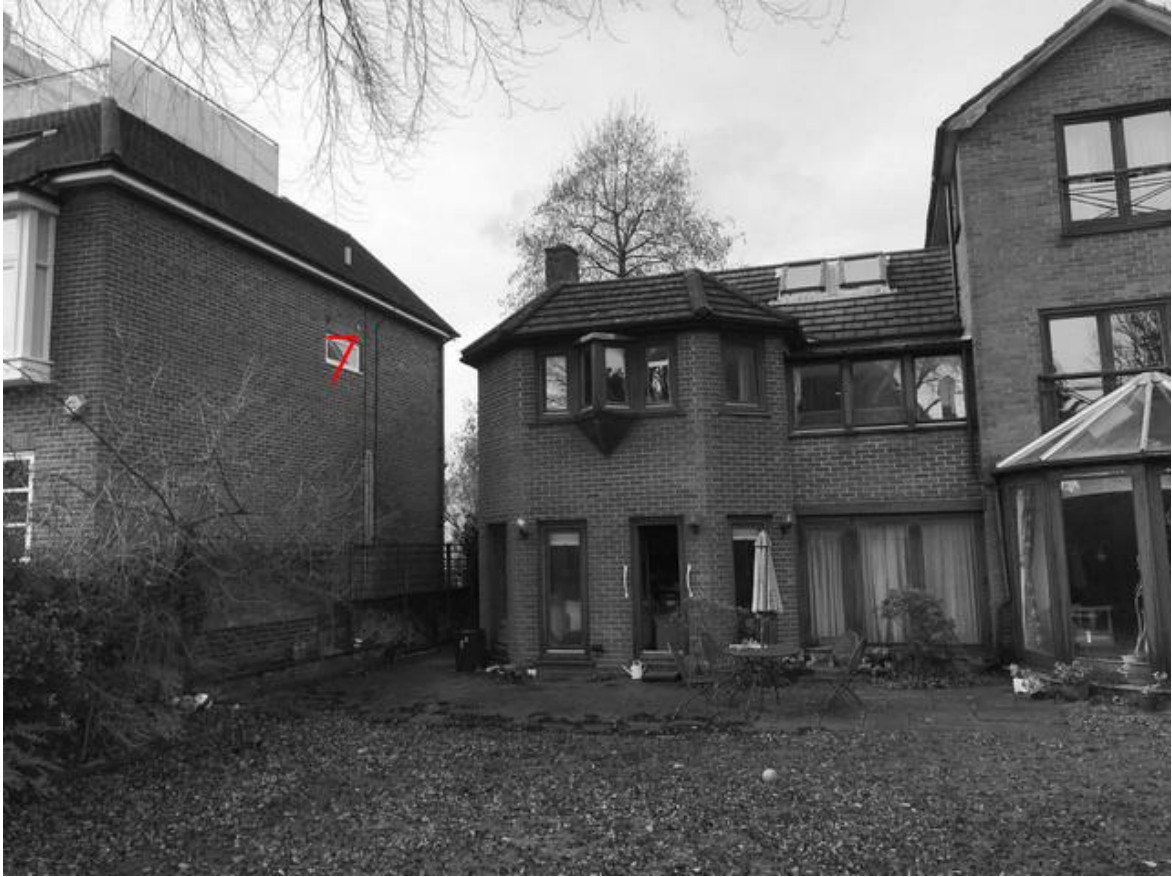
Above – Window 7 at 7-9 Prince Arthur Road
