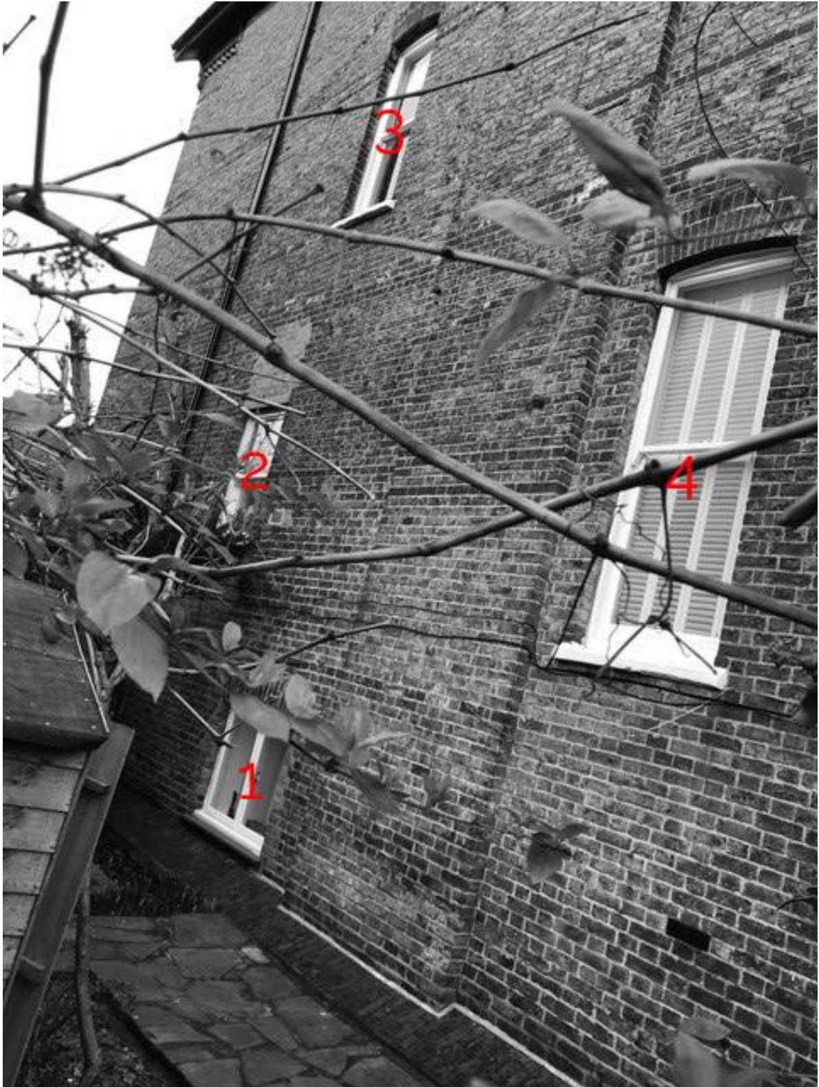
Above – Windows 1 to 4 at 5 Prince Arthur Road
