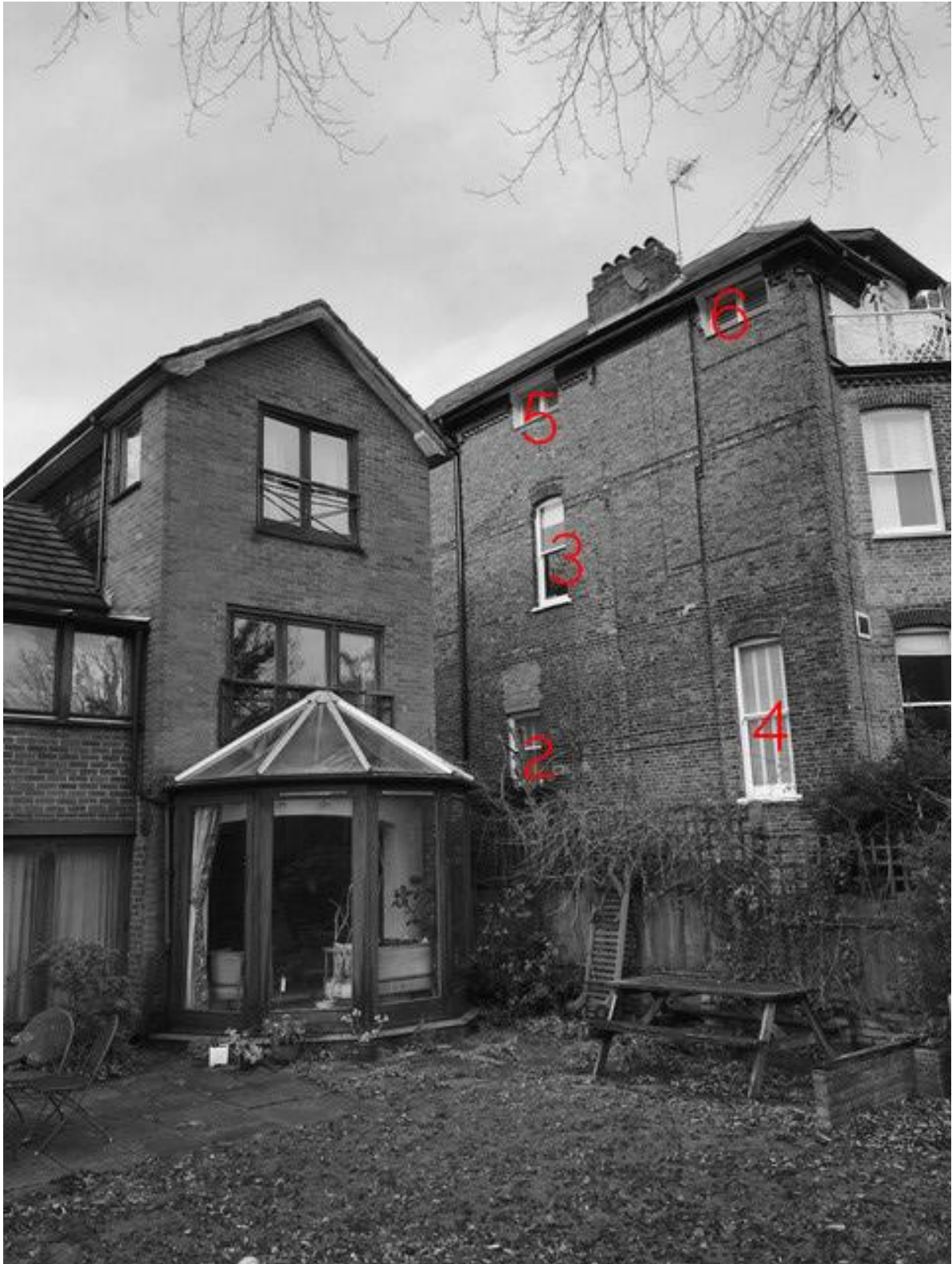
Above – Windows 2 to 6 at 5 Prince Arthur Road
