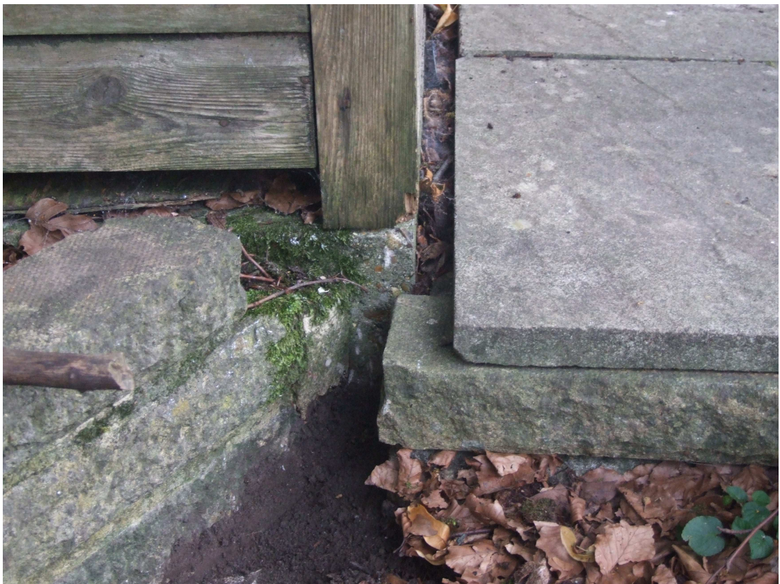
Garden building and lifted paver to show extent of concreting. Present drainage increases the rain shadow effect of the pavers.
