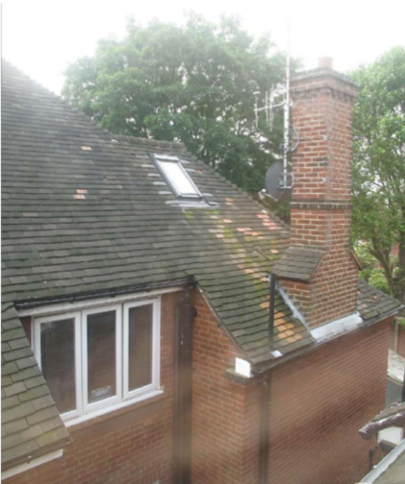
Missing and broken tiles and repairs to 7 Perceval Avenue's roof
