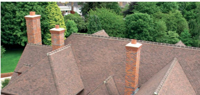
Proposed finish: tile with natural variations in shape and tone, such as Keymer Goxhill handmade plain tiles. This tile is supplied in three different colours so the best match from this or a similar range would be selected after viewing sample panels on site.
