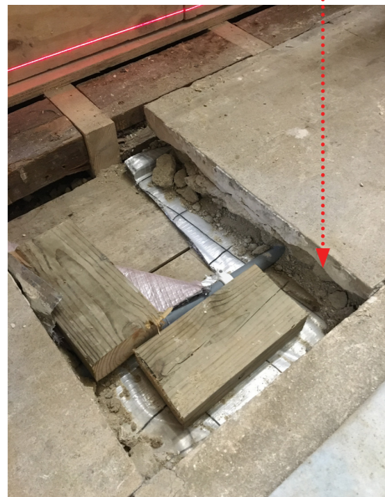
33 Fitzroy Square - Opening Up
