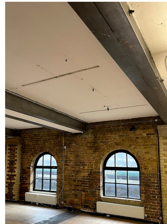
Cast iron columns and beams
