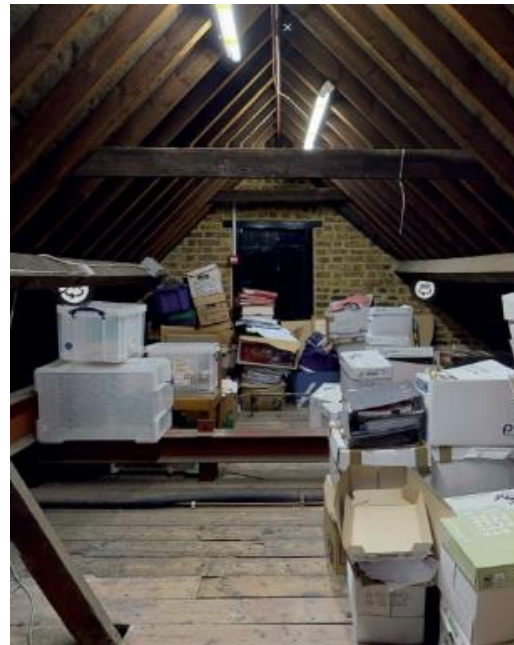
Figure 14: View of the rear attic space showing rebuilt party wall with no.9, modern timber, water proofing membrane and steel work.
