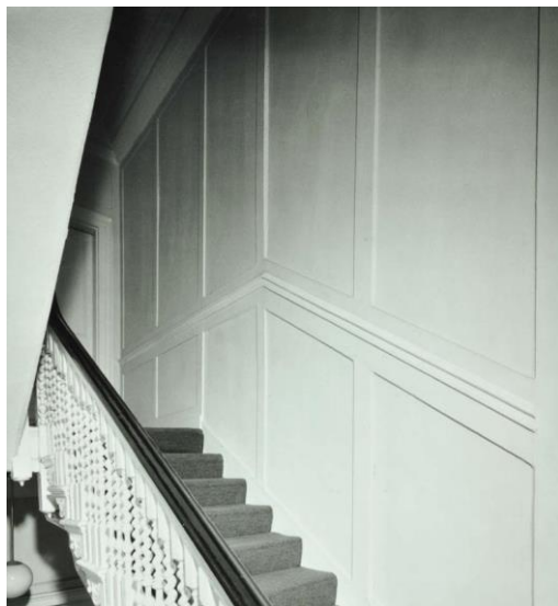
A view of a staircase at 8 Great James Street in 1973 [71858] thought to be taken from first floor to half landing showing the do to the cantilevered WC.
