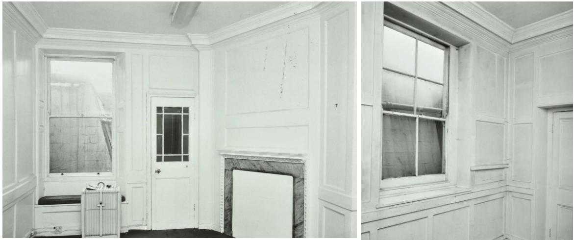
Two views of a ground-floor rear room at 8 Great James Street in 1976 [71889, 71888]
