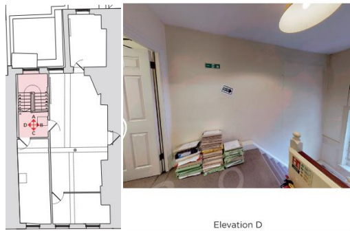
Figure 22: plain plastered landing wall with stepped string at third floor level
