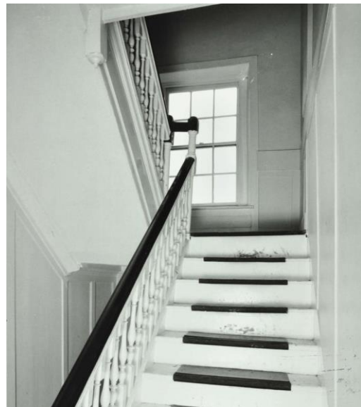
Figure 20: A view of a staircase from 2 nd to 3 rd floor at 8 Great James Street in 1976, [71894]
