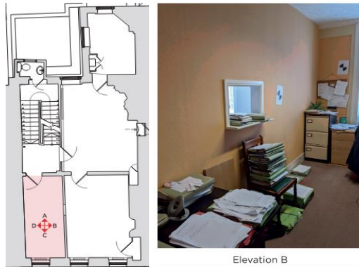
Figure 16: Images showing 2 nd floor front room with modern partition dividing the space
