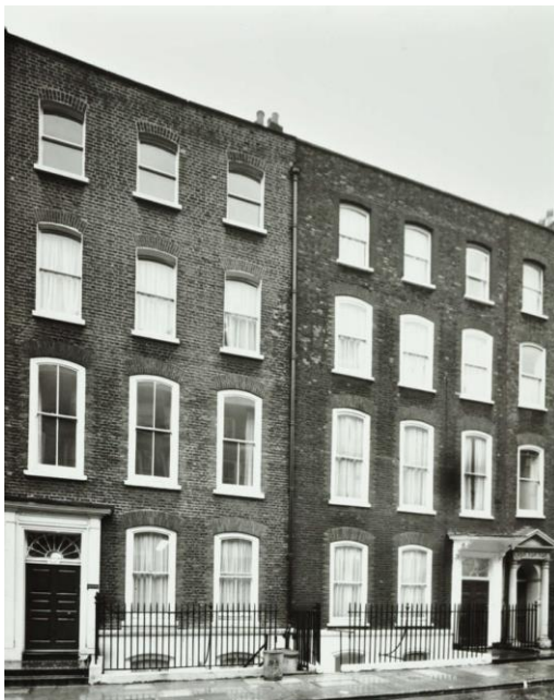
Figure 9: Nos. 7-8 Great James Street in 1969. Panelled doors can be seen and one door has enriched carved bracket carrying hood, both with patterned radial fanlights. Between the houses, lead rainwater heads and lead pipes are
