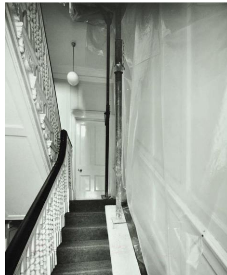
Views of the staircase at 8 Great James Street from ground floor landing to first floor taken in 1973, 3 years before the building was listed. Intriguingly the image show agrow props supporting the flight to 2 nd floor.
