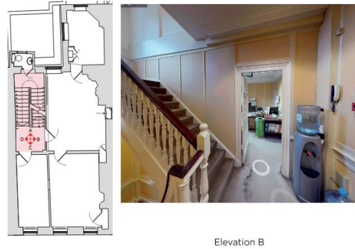
Figure 17: Image showing 2 nd floor landing and modern flight of stairs to the 3 rd floor.
