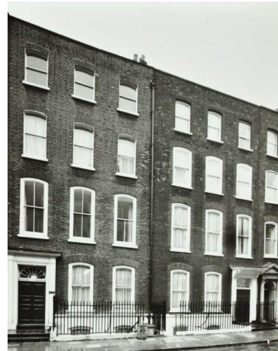
Figure 3: Nos. 7-8 Great James Street in 1969. Panelled doors can be seen and one door has enriched carved bracket carrying hood, both with patterned radial fanlights. Between the houses, lead rainwater heads and lead pipes are visible. Iron railings are seen by the basement with finials on corners. [© LMA Collage Collection, image no. 71770]
