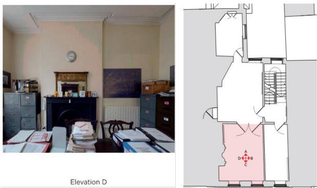
Figure 14 (top) and 15 (above) showing current first floor front rooms with no panelling, later cornice, lowered ceiling and modern fire place
