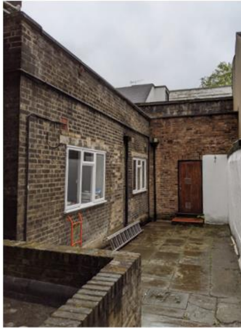
Figure 20: Existing rear extension to be replaced
