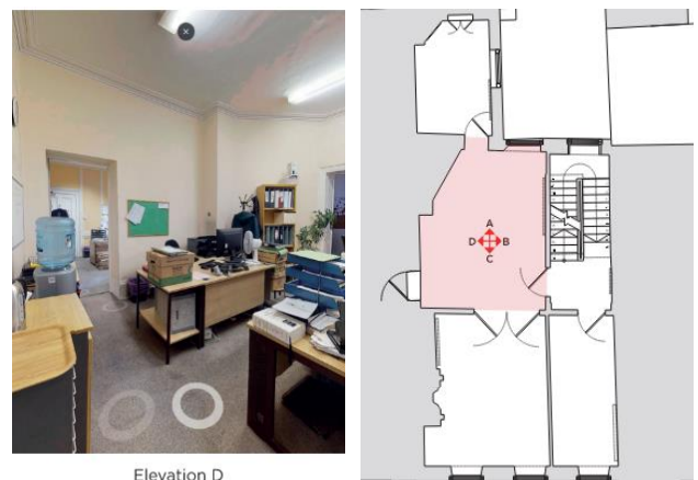
Figure 16 – First floor rear room with modern plaster walls, small plaster cornice, door cojoining no.8 Great James Street and no fireplace.
