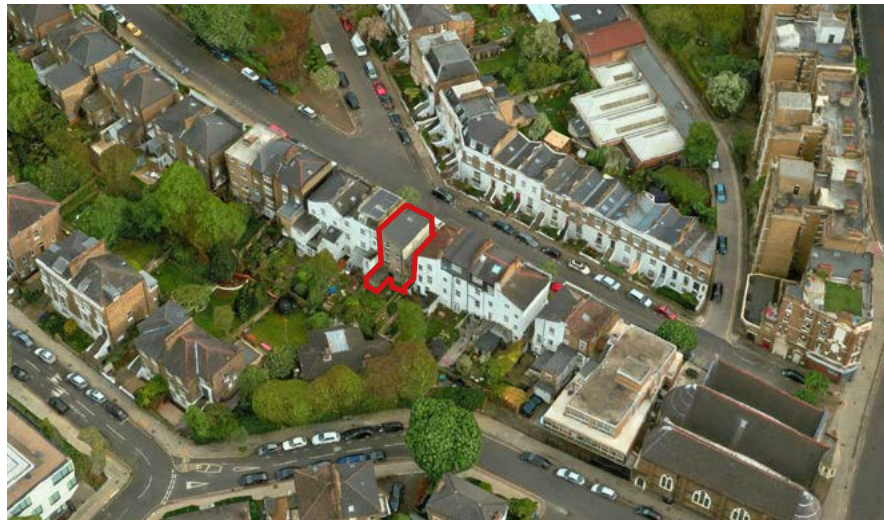
Aerial view from the Northwest Source: Apple Maps
