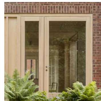
2 Timber framed glazing
