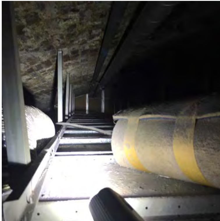
Photograph 7 – Intact brickwork in railway arches
