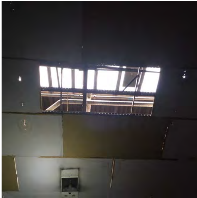
Photograph 5 – Holes in ceiling showing skylight and roof structure
