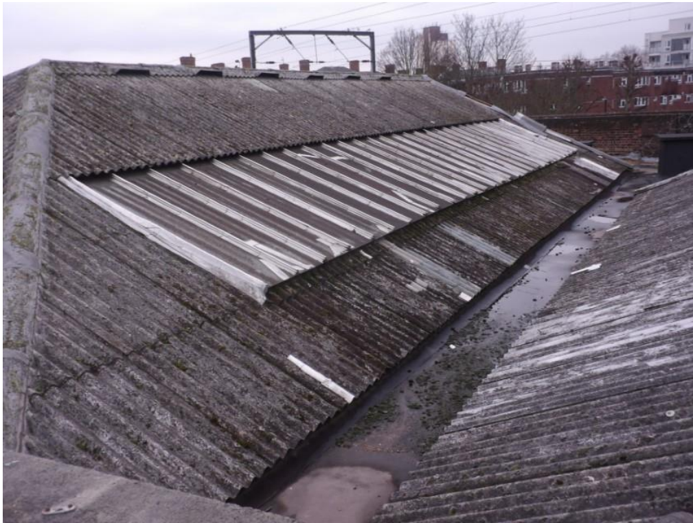
General view of pitched roof areas with corrugated asbestos sheeting.
