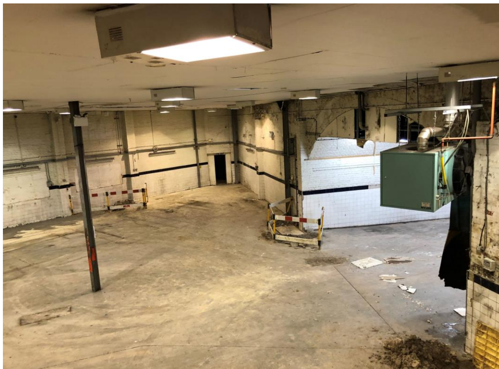
General view of secondary warehouse area (zone 4).
