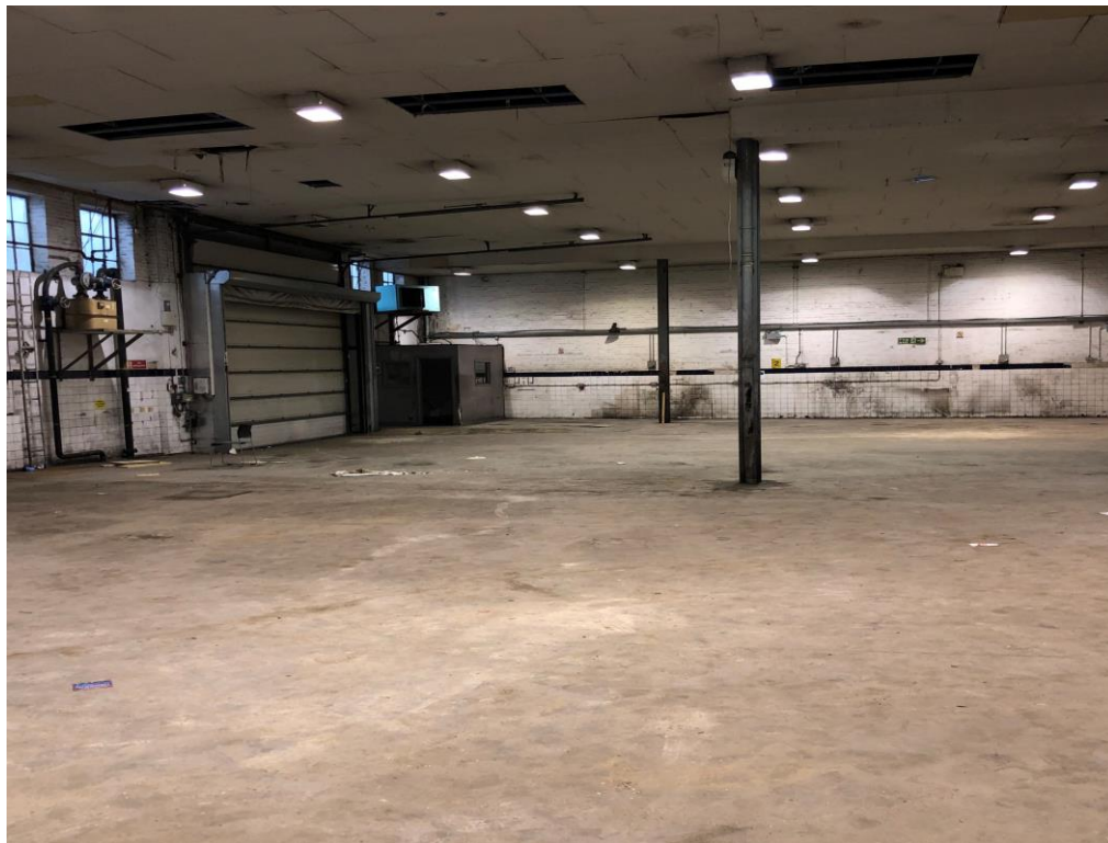
General view of primary warehouse area (zone 1).
