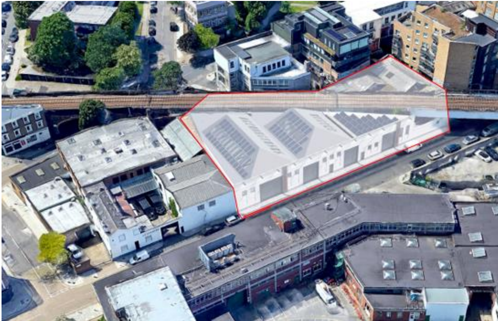
Aerial view of site (highlighted)
