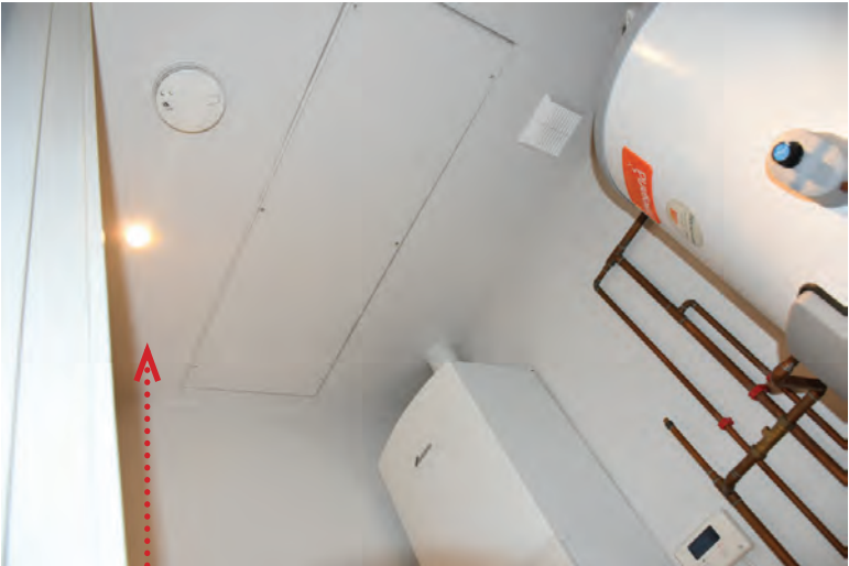
U1 Route for New Vertical Ducts
