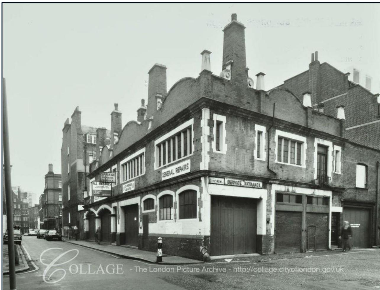
**Figure 5.** A photograph from 1978 looking south east at the corner of John's Mews and Northington Street. The Site is seen here as a closed and for sale Goodliffe Garages Limited. A number of external alterations had been made by this time to accommodate its operation, including roller shutter openings (seen to the right), which allowed access to a ramp down to a basement.
