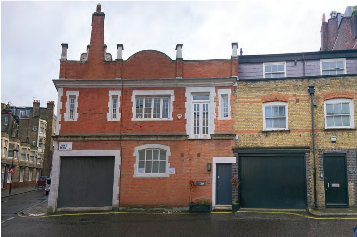
Site photo along John's Mews
