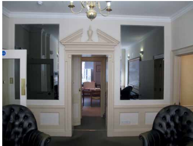
Photo 01 Room FR02. The wall between FR02 and corridor to FR08 has been replaced with a late C20 th postmodern interpretation of Georgian architecture, including an elaborate timber doorcase entry and panelling and tinted mirror panels.
