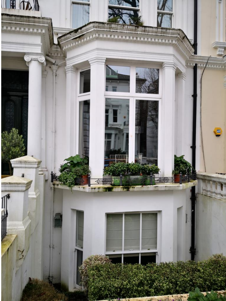
Existing lowered garden area at front of No. 31
