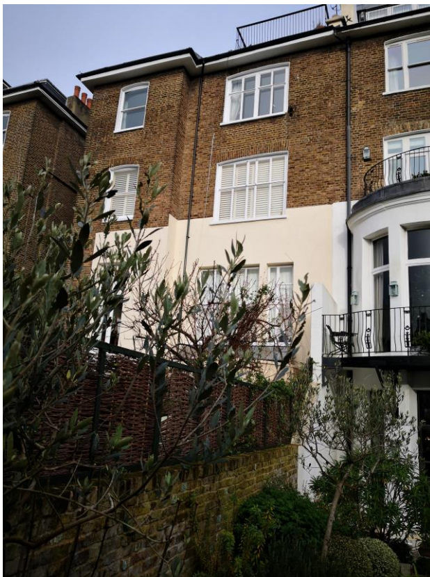
Adjoining property of No. 29, showing lack of symmetry to pair of houses
