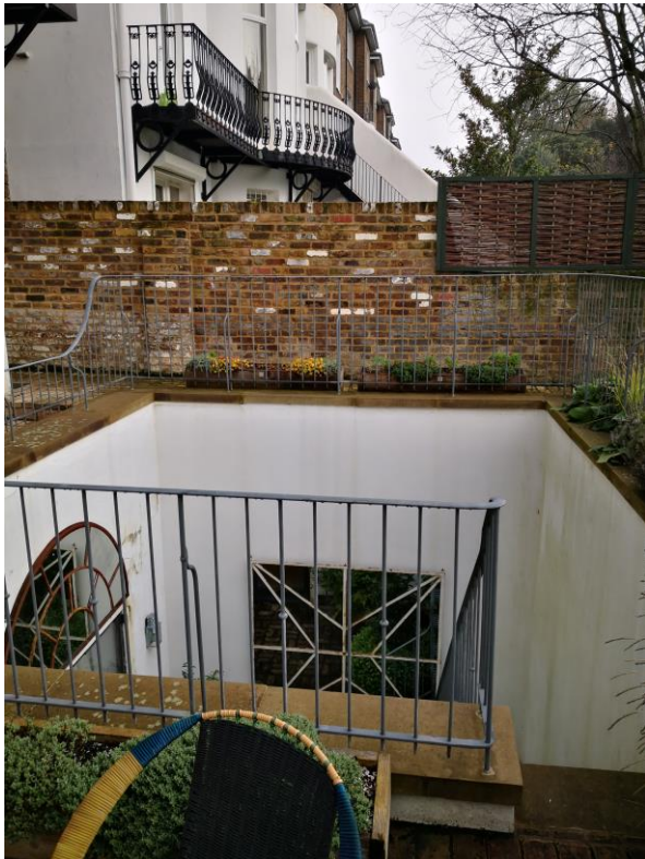
Existing lightwell to No. 31, to be covered
