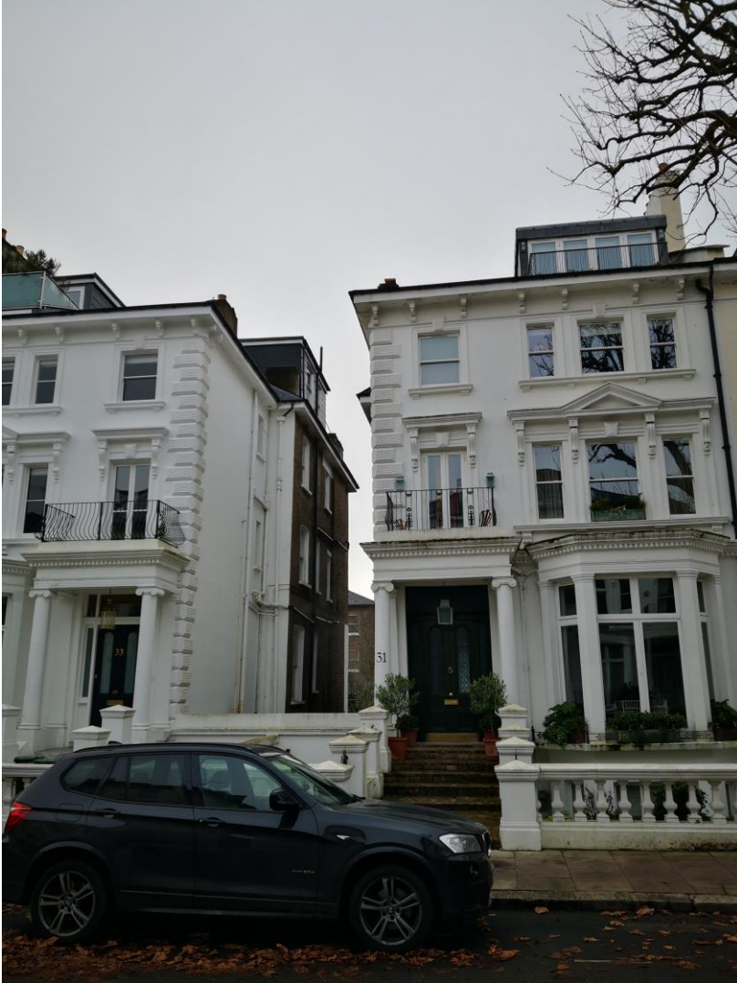
No., 31 from the street, with side dormer to No. 33 visible
