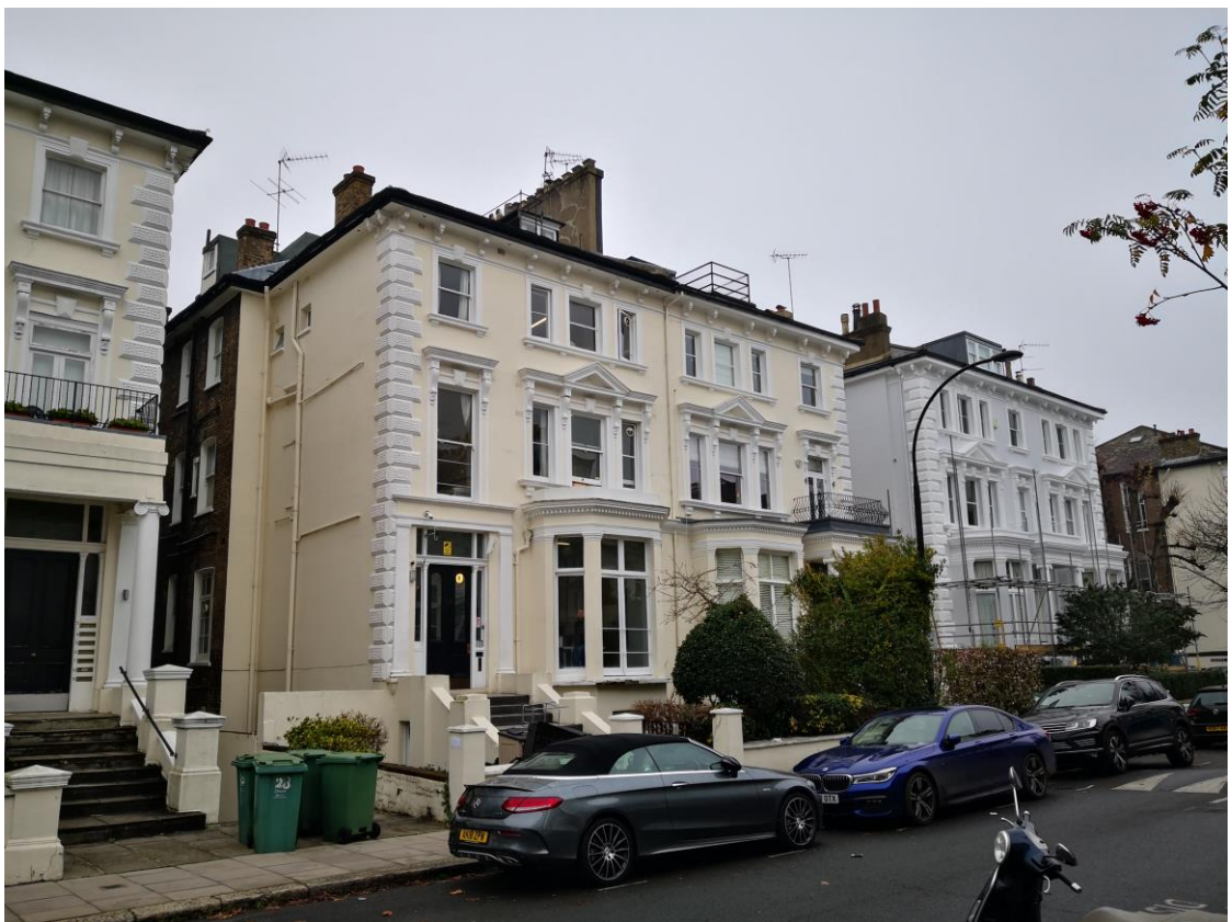
Dormers and additions to properties along Belsize Park Gardens
