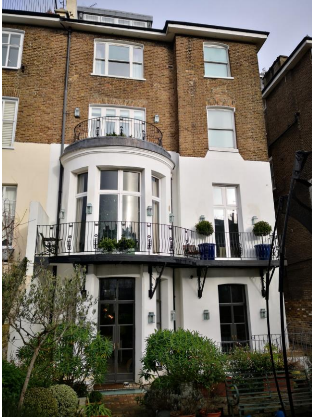
Rear of No. 31
